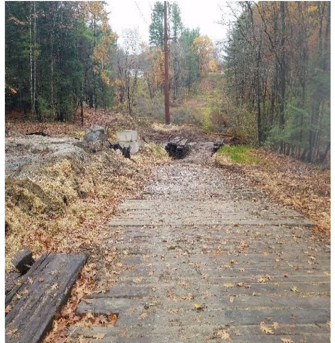
Fig 6: Access to Str. 28 beginning to be removed. Viewing north. (10-28-19).
