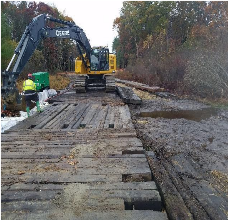
Fig 5: Beginning to remove stream bypass in Knights Brook. Viewing west. (10-28-19).
