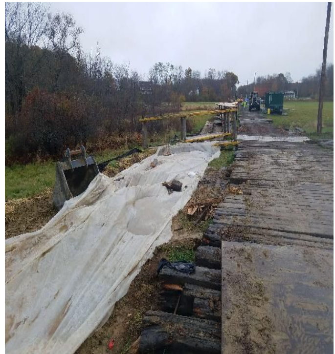
Fig 4: Exposed soils covered with plastic at Frink farm. Viewing east. (10-28-19).
