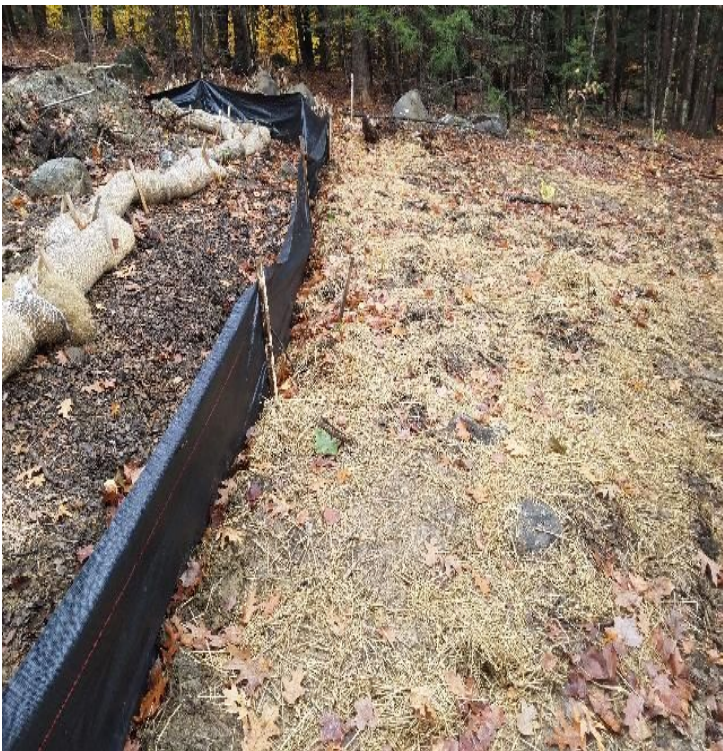
Fig 7: Silt fence downslope of Str. 29. Viewing west. (10-28-19).
